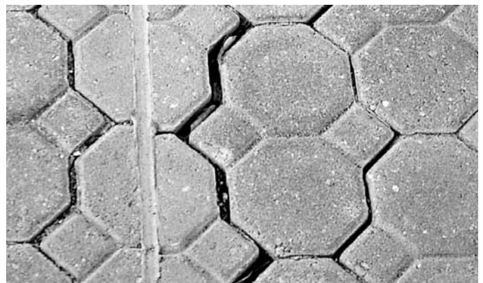
Figure 12. An absence of edge restraints and use of a sealant in this construction joint caused the pavers to shift and open their joints on both sides of the sealant.
